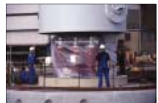
The switchgear and transformer was placed on top of the concrete foundation just before placement of the lower part of the tower.
