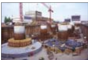
Casting of foundations in an old dry dock in the former B&W Shipyard. The dry dock could exactly hold 20 foundations. The shape of the ice cone is inspired from the hull of a ship and popularly known as 'the Tulip'.
