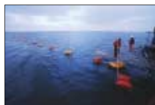
Placement of submarine cables. The cables are carefully placed on air cushions and floated to the final position. The air is released from the cushions one by one and a diver on the bottom secures the correct position.
