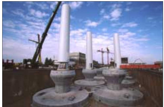
The switchgear and transformer was placed on top of the concrete foundation just before placement of the lower part of the tower.
