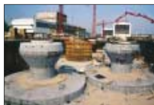
Casting of foundations in an old dry dock in the former B&W Shipyard. The dry dock could exactly hold 20 foundations. The shape of the ice cone is inspired from the hull of a ship and popularly known as 'the Tulip'.
