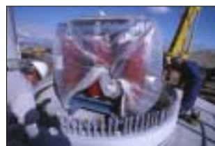
The switchgear and transformer was placed on top of the concrete foundation just before placement of the lower part of the tower.
