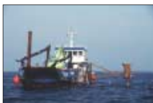
The rock cushion is prepared for the foundation.
