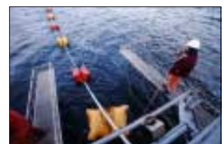
Placement of submarine cables. The cables are carefully placed on air cushions and floated to the final position. The air is released from the cushions one by one and a diver on the bottom secures the correct position.
